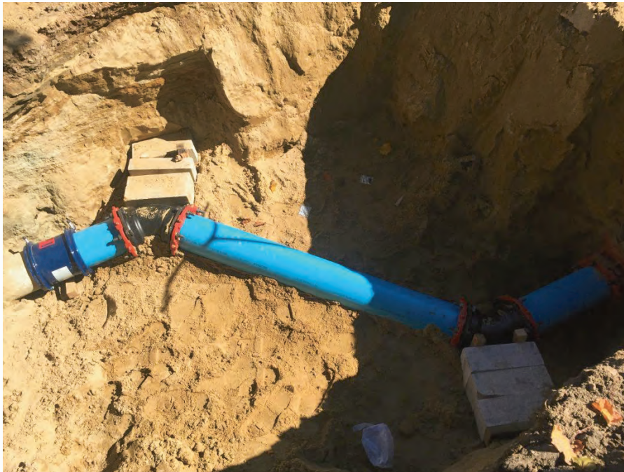
Connection to existing Main on Fulton St. @ Garden St.
